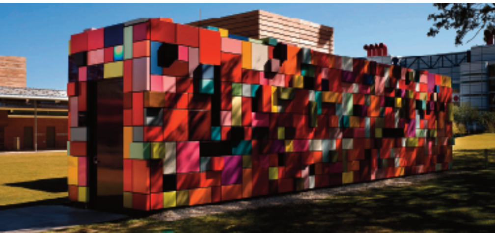
Below: Synchronicity of Color—Red , 2008. Bottom: Synchronicity of Color—Blue , 2008. Painted aluminum boxes mounted on aluminum panels, mounted to metal hat-channels on a concrete building, 2 elements, 12.5 x 9.5 x 50.5 ft. each.
